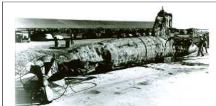
This is a Japanese, Ha-19 “Type A, Midget submarine” sank by the destroyer USS Monaghan on December 7, 1941. The damage to the submarine’s hull is from depth charges and ramming. This is the same type of a two-man, “Midget” submarine that fired two torpedoes at the USS St. Louis as it left Pearl Harbor. The Japanese transported the Midget submarine aboard a larger I-24 submarine, to the waters off Pearl Harbor, where it was released for the attack. They launched five such Midget submarines for the attack on Pearl Harbor.
